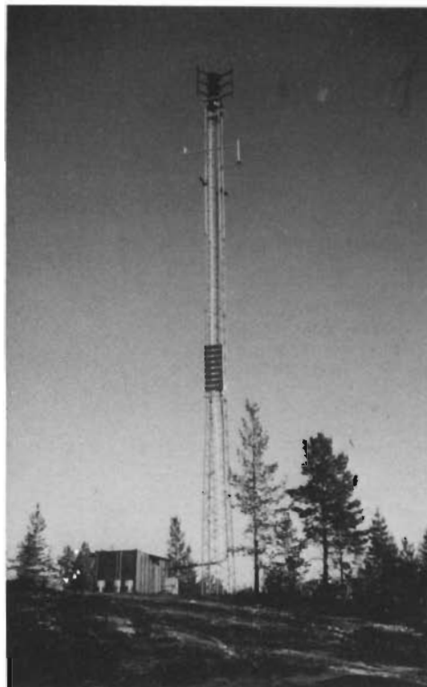
Fig. 8 The ERIGEN powered radio repeater for the Swedish Railways.
